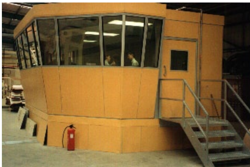
Figure 12 A noise refuge and control room
