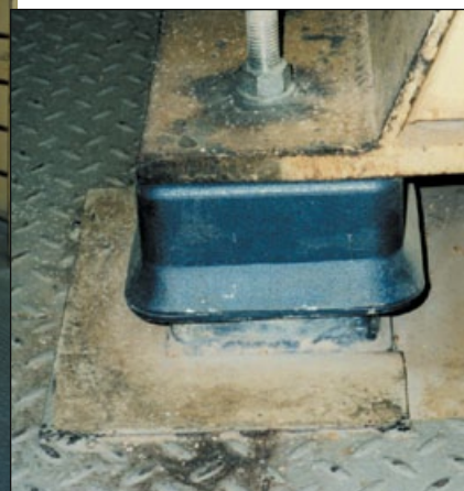
Figure 16 Detail of anti-vibration mount
